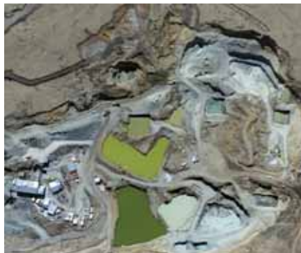
Top Liqhobong Plant
